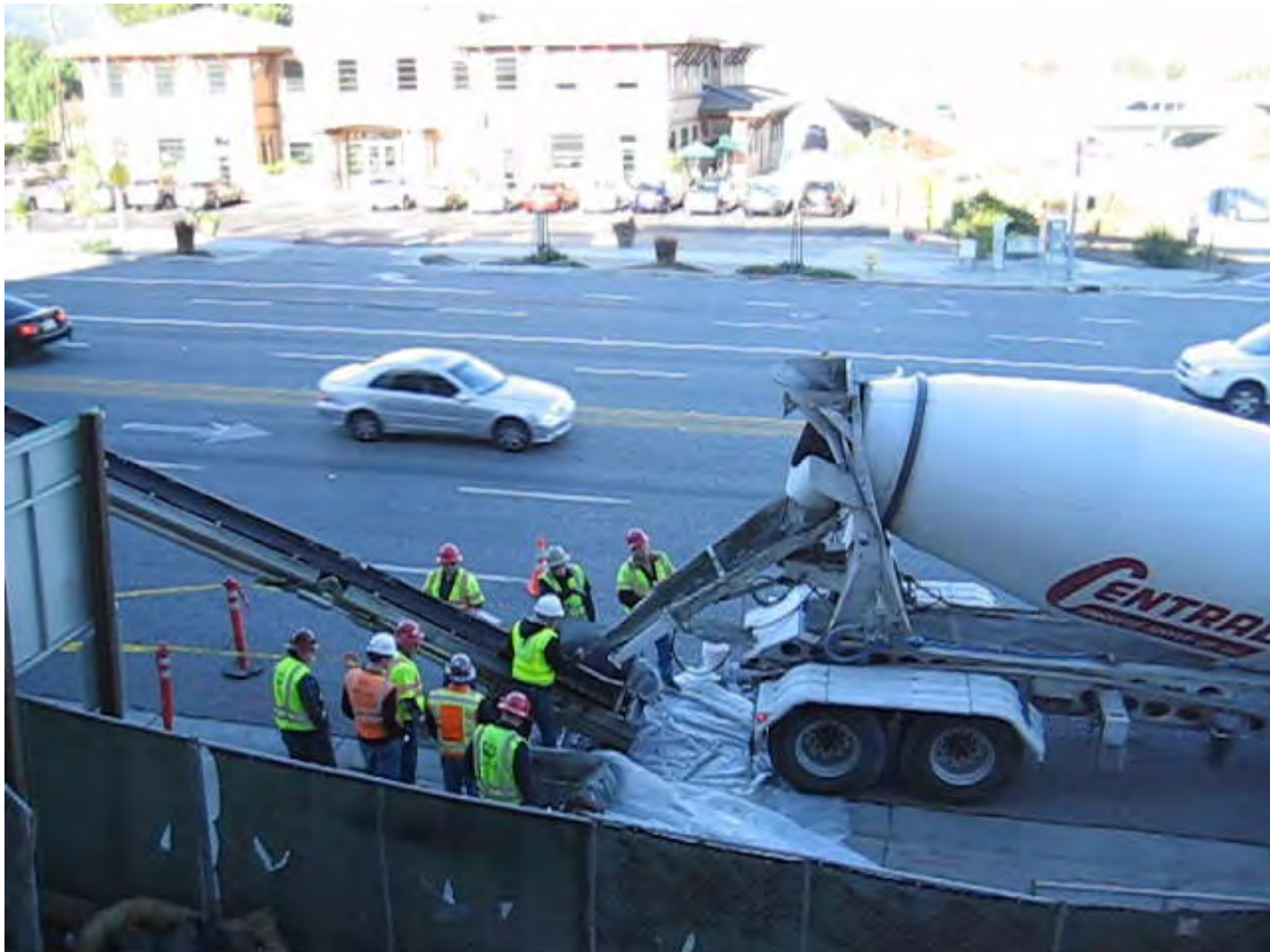
Placement High Density Concrete supplied by Central Concrete
