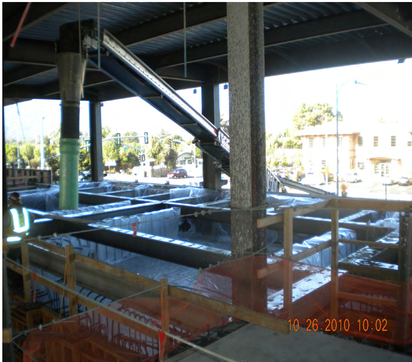
Test run: Checked maximum free-fall of aggregate
